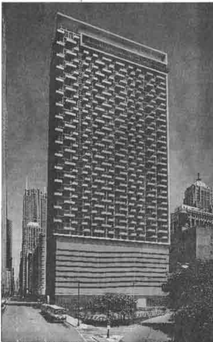
Condos begin at $185,900 at 235 Van Buren, a high-rise in the Financial District on the southern edge of the Loop.
